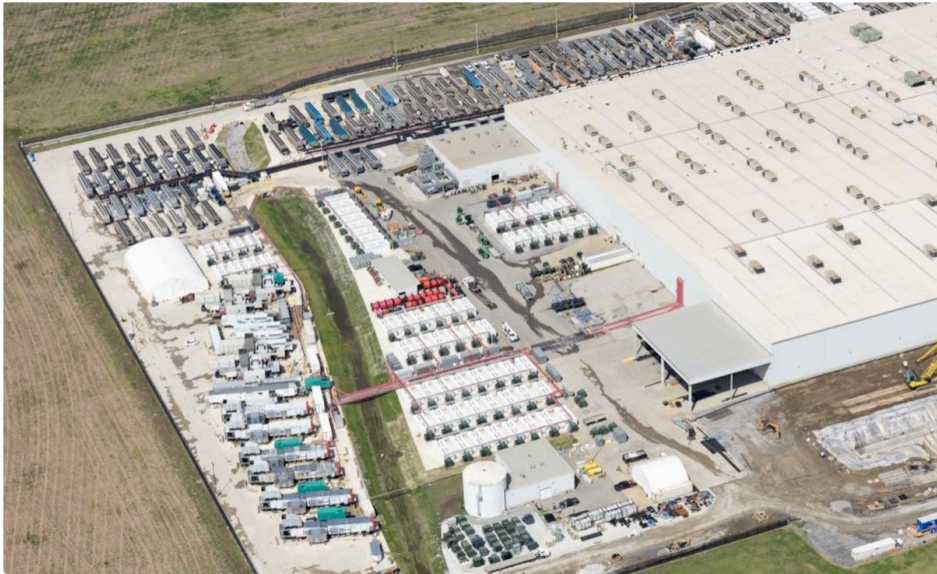
xAI Colossus Data Center, Memphis, TN
