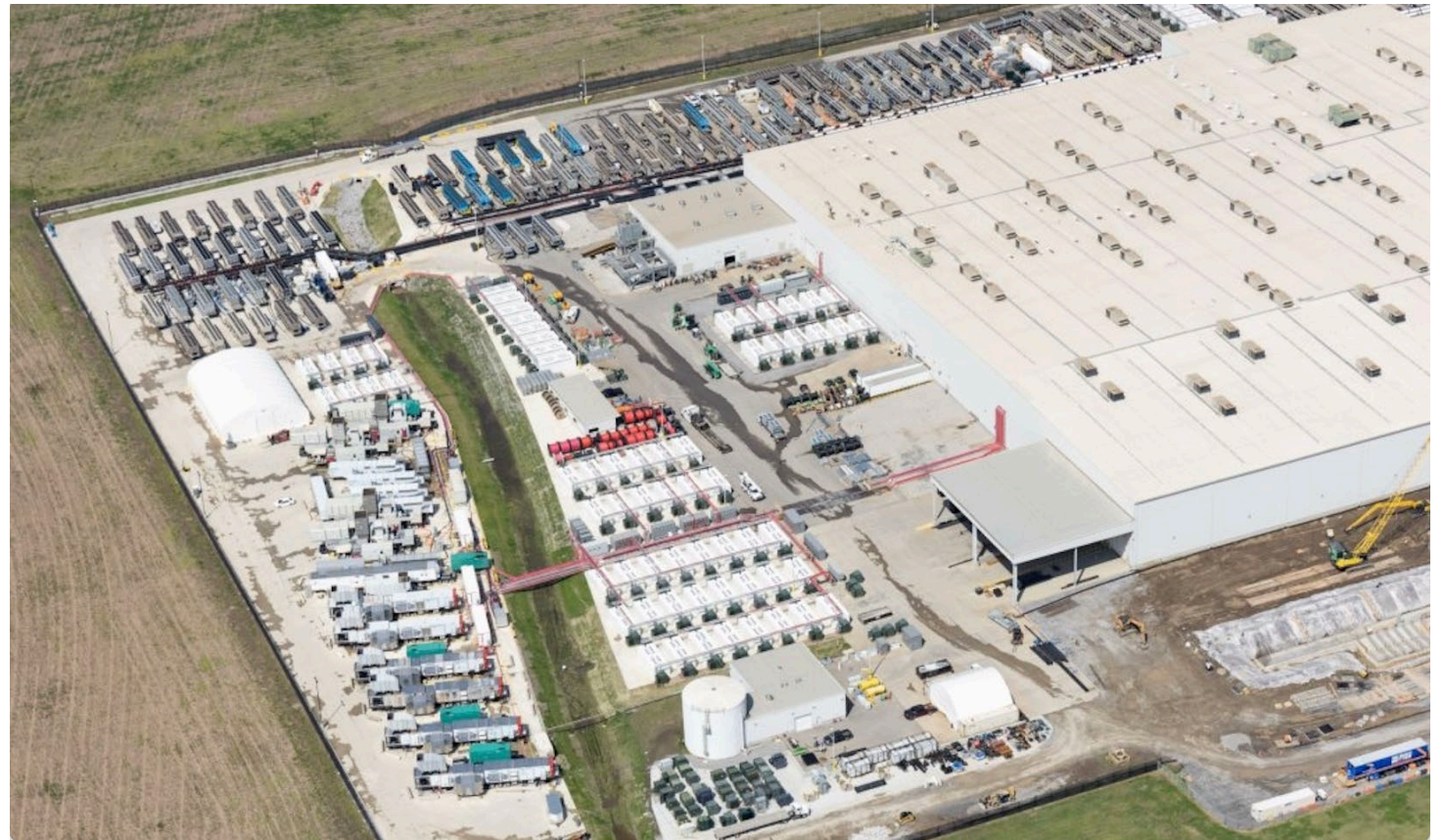
xAI Colossus Data Center, Memphis, TN
