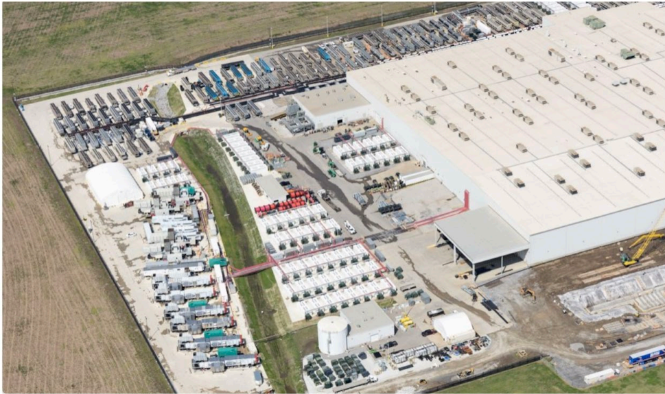
xAI Colossus Data Center, Memphis, TN
