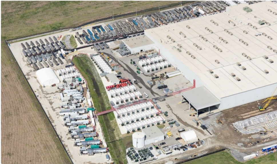
xAI Colossus Data Center, Memphis, TN
