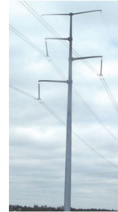
Single-circuit bundled conductor
