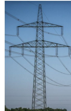
Double-circuit bundled conductor
