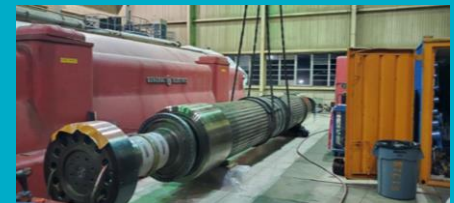
Low-pressure turbine rotor blast cleaning process
