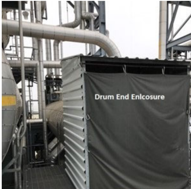
Hardened wind break needed on upper levels
