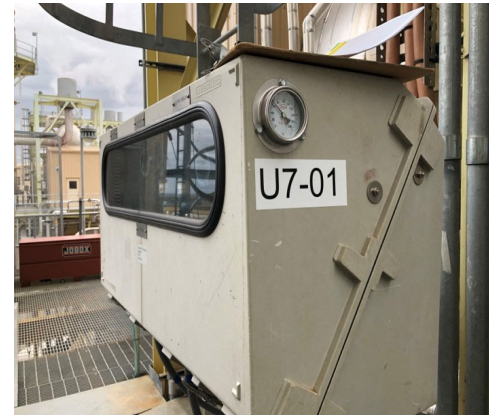
Transmitters enclosure with temperature gauge for monitoring inside temperature
