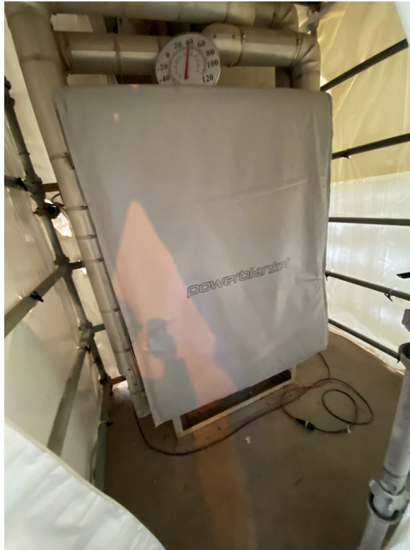
Using shrink wrap and zippers for enclosures. We also found that labeling the enclosures was helpful for the contractors.
