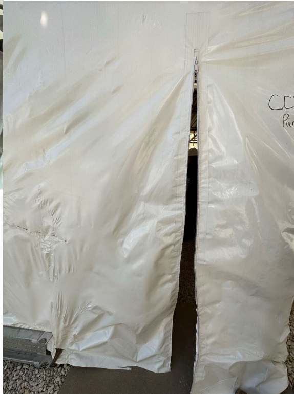
Using shrink wrap and zippers for enclosures. We also found that labeling the enclosures was helpful for the contractors.
