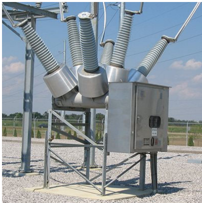
Local Pressure Gauge on SF6 Insulated Breaker
