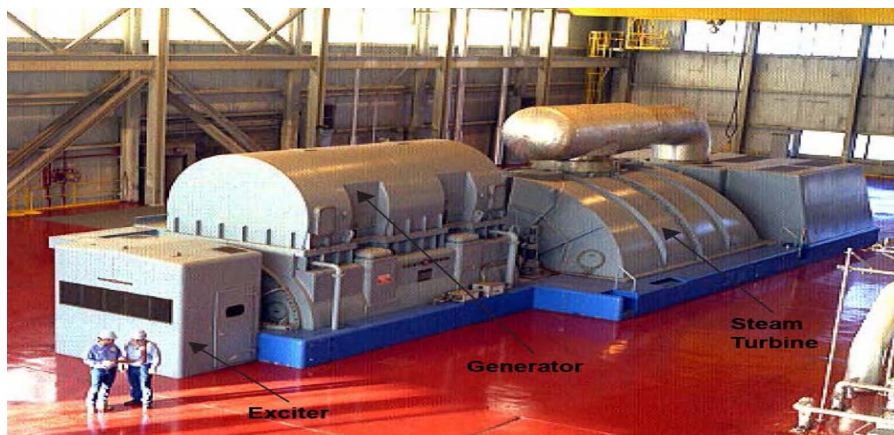
Figure 7: Three-phase power generator (Electric Power Research Institute)
