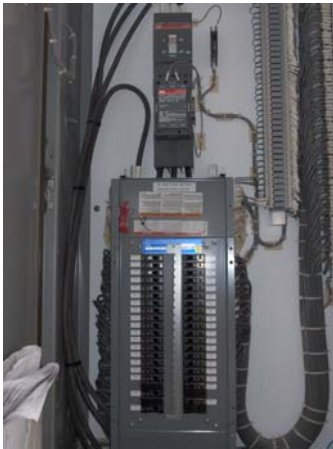
Figure 1: Freeze Protection Panel Interior
