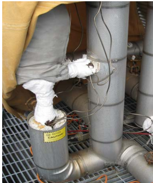
Figure 4: Insulated Piping with Heat Tracing
