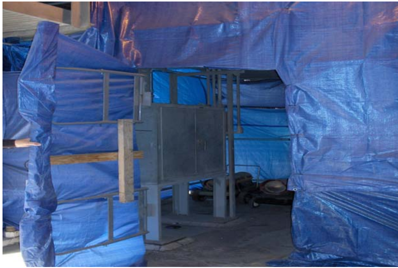
Figure 7: Temporary windbreak created with scaffolding and tarpaulin
