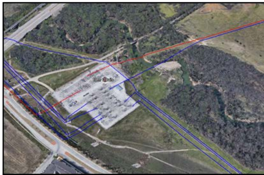
Ben Davis Substation located in Flood Way
