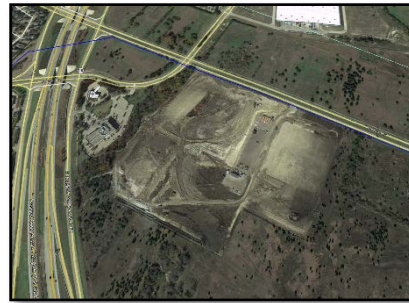
Construction of new Data Center
