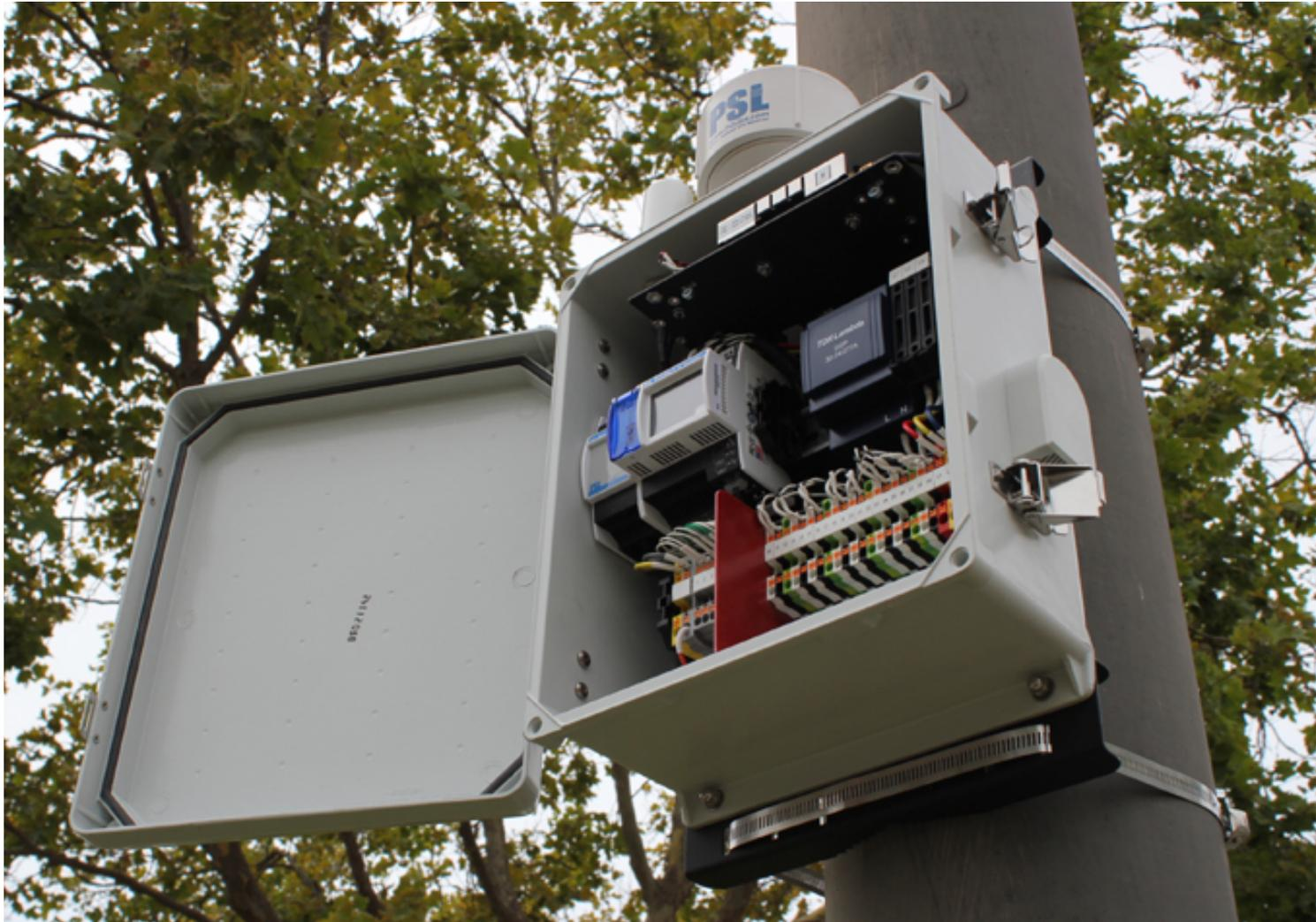
Sample utility polemount installation of  $\mu$ PMU including GPS receiver, modem and antenna
