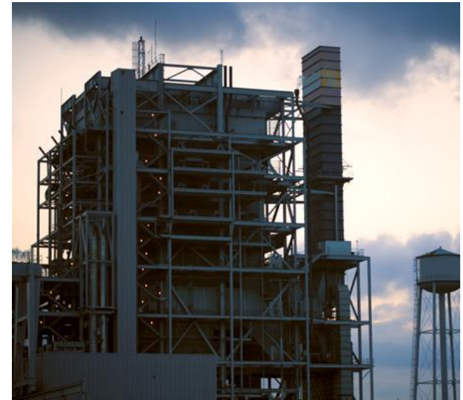
NRG Texas Power Photo
