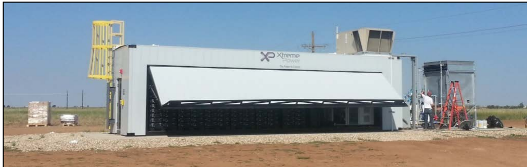
Figure 82. BESS Installed at the Reese Technology Center
