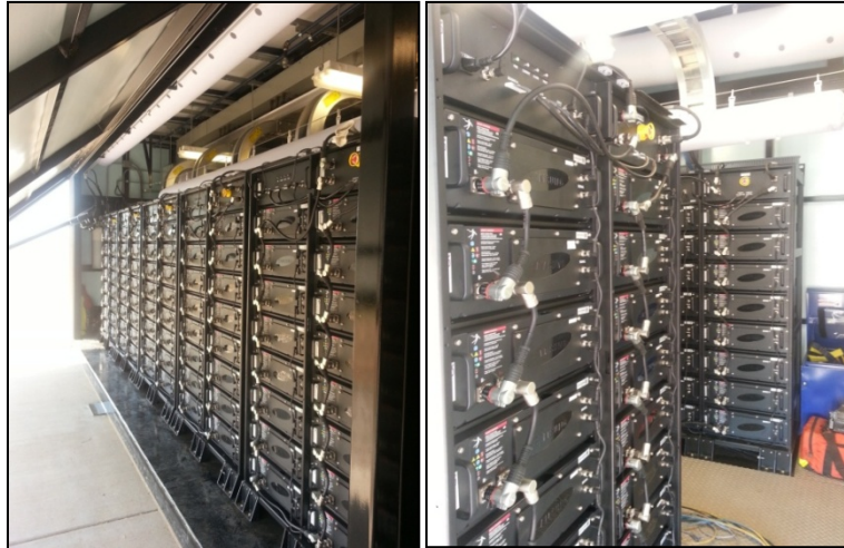
Figure 10. Racks of Batteries within the BESS Container
