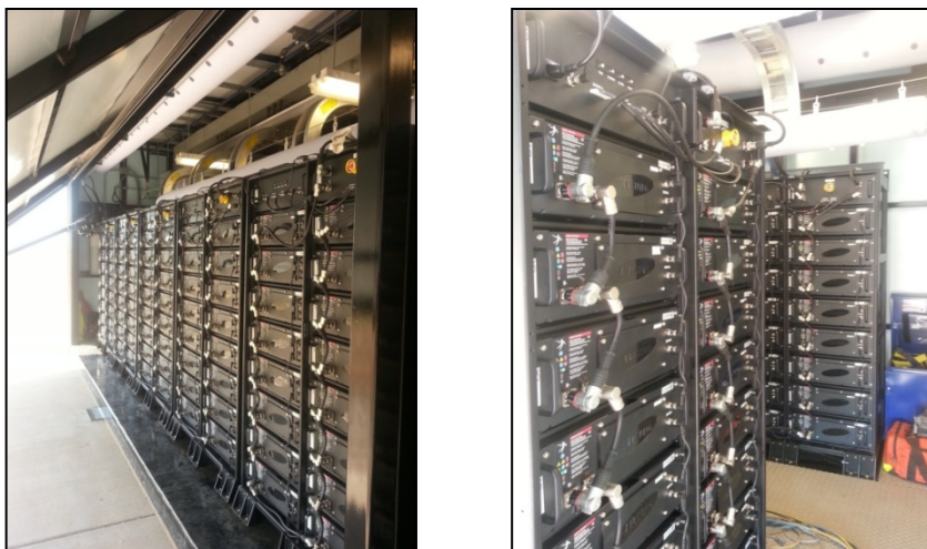
Figure 83. Racks of Batteries within the BESS Container
