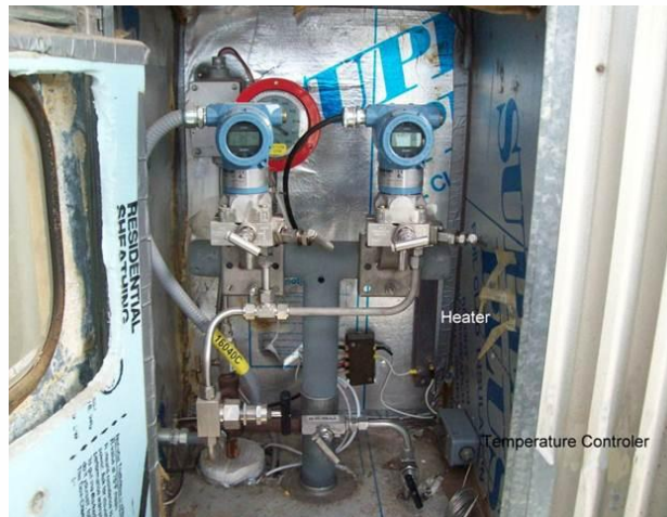
Temporary (winter months only) enclosure to protect boiler drum level critical transmitters
