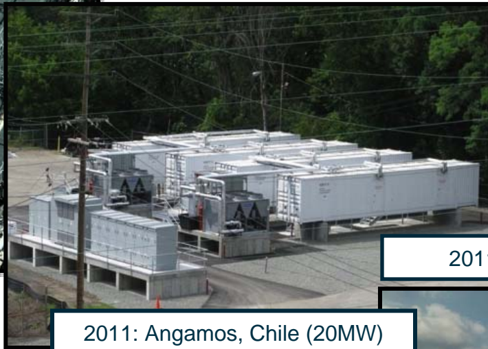
2010: Johnson City, NY (8MW Phase 1)
