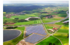
Muehlhausen, GERMANY, 6 MW
