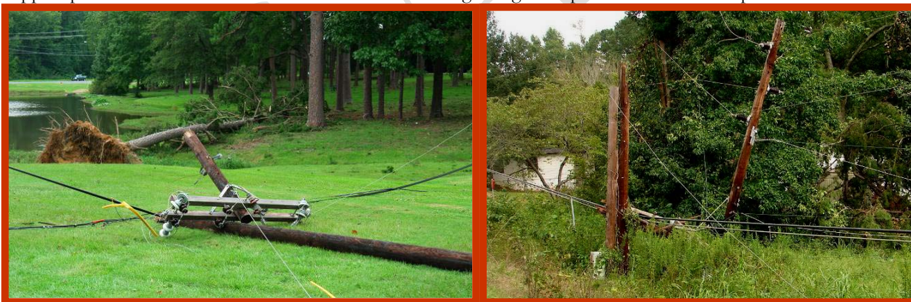
The majority of damage was caused by high wind and trees falling into the lines. ONCOR replaced 658 poles in total.
