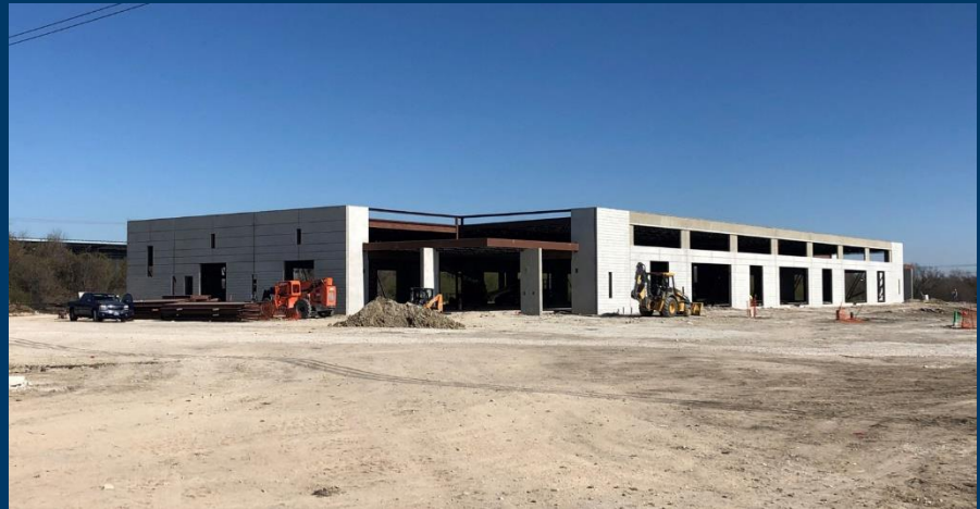
New ERCOT Austin Met Center facility as of mid-January
